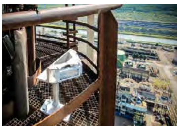
FRANCE, Oil and Gas Chimney
